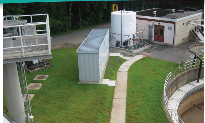
The WRRF in Ridgewood, NJ began receiving fats in 2013 for biogas production at the facility. The original 10,000-gallon capacity was expanded to 30,000 gallons.
